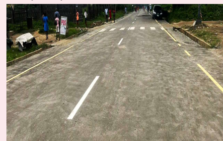
CONSTRUCTION OF 1.2KM UMUOKOMIRI ROAD (EXPRESS TO OBEHIE ROUND ABOUT), UKWA WEST LGA
