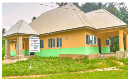
CONSTRUCTION OF ETI COMMUNITY HALL, UKWA EAST LGA
