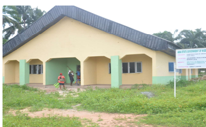
CONSTRUCTION OF UMUEZEGU HALL, NSULU, ISIALA NGWA NORTH LGA
