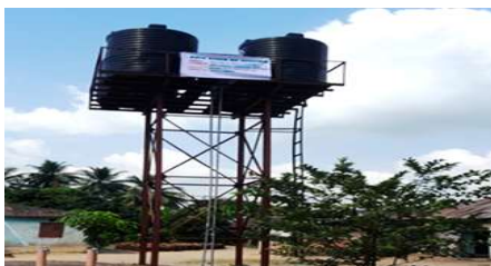
DRILLING OF WATER BOREHOLE AND RETICULATION AT OHANDU AUTONOMOUS COMMUNITY OHANDU NDOKI, UKWA EAST LGA
