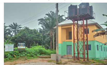
CONSTRUCTION OF AMAORJI UMENKWUOHU CIVIC HALL OBEAKU NDOKI, UKWA EAST LGA
