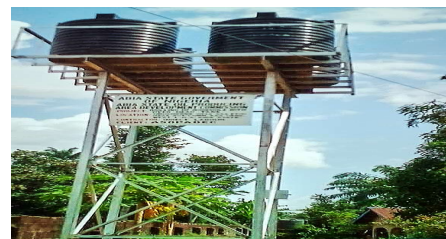
CONSTRUCTION OF BOREHOLE AT UMUADIENWE, UKWA WEST LGA
