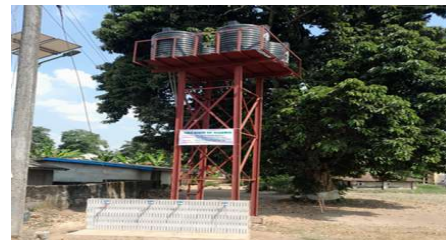
DRILLING OF WATER BOREHOLE WITH TANK AND STANCHION AT AKANU NDOKI VILLAGE IN IKWOORIE ATO IN NDOKI, UKWA EAST LGA
