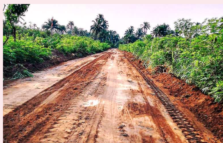
GRADING OF 8KM ROAD AT OWO ASA UMUADIEWE, UKWA WEST LGA
