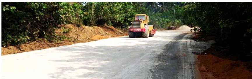
REHABILITATION OF SELECTED UMUNTEKE INTERNAL ROADS UKWA WEST LGA (3.3 KM)
