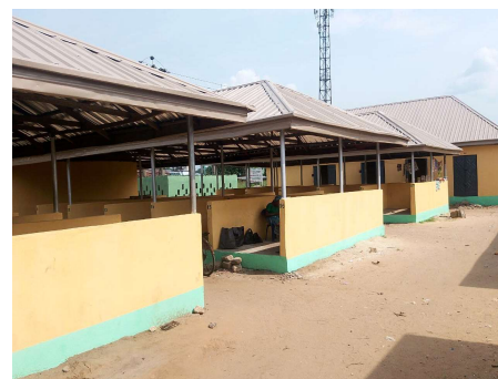
CONSTRUCTION AND RECONSTRUCTION OF MARKET STALLS ARE AHIA ORIE, OBOKWE, UKWA WEST LGA
