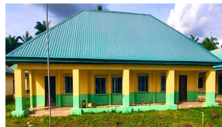
CONSTRUCTION OF COMPUTER HALL AT MBATO SECONDARY SCHOOL UMUNGALAGU NVOSI AUTONOMOUS COMMUNITY, ISIALA NGWA SOUTH LGA
