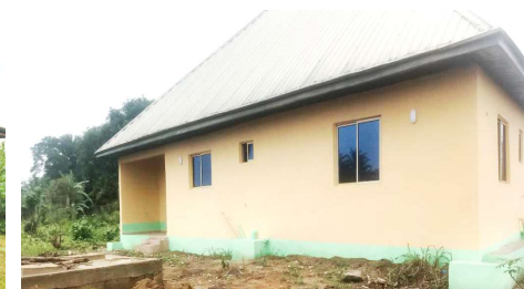
CONSTRUCTION OF A THREE BEDROOM FLAT FOR NURSES AT COTTAGE HOSPITAL OWAZA, UKWA WEST LGA
