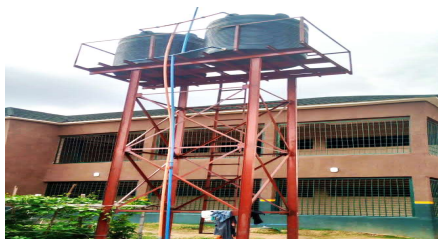
DRILLING OF MOTORIZED BOREHOLE AT CUSTODIAL CENTRE UMUAHIA NORTH LGA
