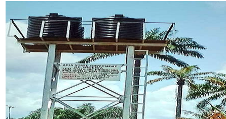
DRILLING OF WATER BORE HOLE AT UMUEZEKE OBIINGWU RD ASA NORTH, UKWA WEST LGA
