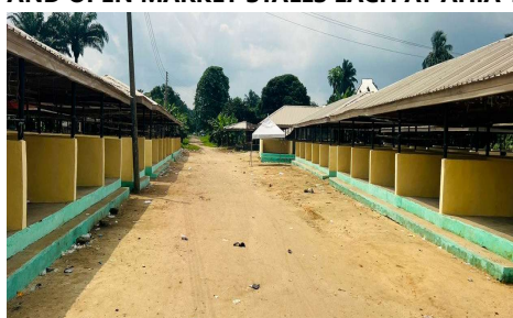
CONSTRUCTION OF FOURTEEN (14) BLOCKS OF TEN (10NOS) OPEN MARKET STALL AND RENOVATION OF TWO BLOCKS OF TEN (10NOS) OPEN MARKET STALLS AT AHIA ORIE UMUJIOHA OBUZOR ASA COMMUNITY MARKET, UKWA WEST LGA
