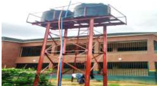
DRILLING OF MOTORIZED BOREHOLE AT CUSTODIAL CENTRE UMUHIA NORTH LGA
