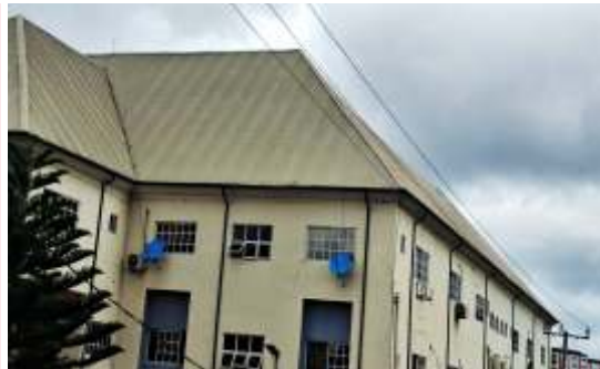
RE-ROOFING OF ASOPADEC OFFICE COMPLEX, UMUAHIA NORTH LGA
