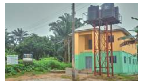
CONSTRUCTION OF AMAORJI UMENKWUOHU CIVIC HALL OBEAKU NDOKI, UKWA EAST LGA
