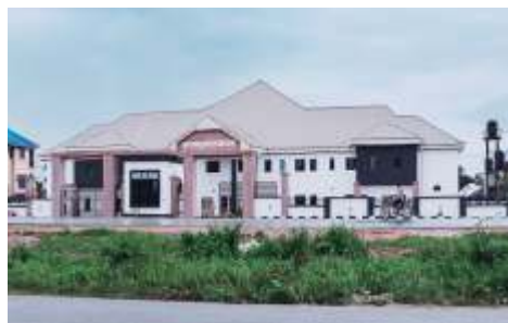
CONSTRUCTION OF ASA CIVIC CENTER, OBEHIE, UKWA WEST LGA
