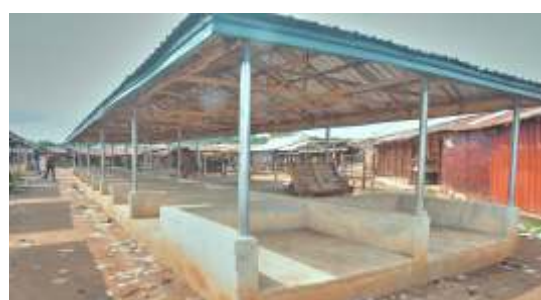
CONSTRUCTION OF OPEN MARKET STALLS AT AHIA ORIE AMAPU NTIGHA MARKET, ISIALA NGWA NORTH LGA
