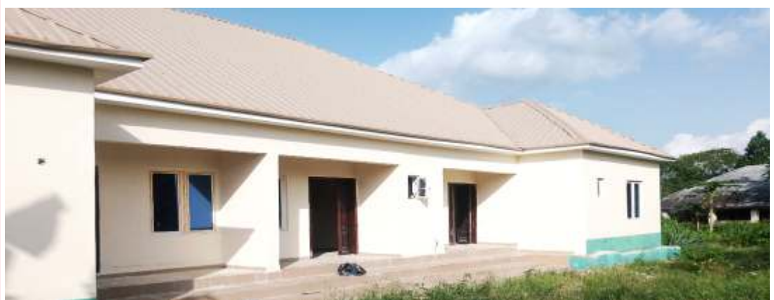
CONSTRUCTION OF RESIDENTIAL BLOCK OF THREE (3) FLATS AT OBEHIE HEALTH CENTRE, UKWA WEST LGA
