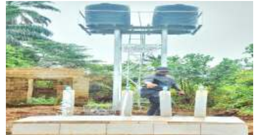
CONSTRUCTION OF BOREHOLE AT UMUINWERE, OBOKWE, UKWA WEST LGA
