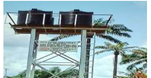
DRILLING OF WATER BORE HOLE AT UMUEZEKE OBINGWU RD ASA NORTH, UKWA WEST LGA
