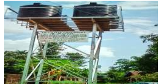
CONSTRUCTION OF BOREHOLE AT UMUADIENWE, UKWA WEST LGA
