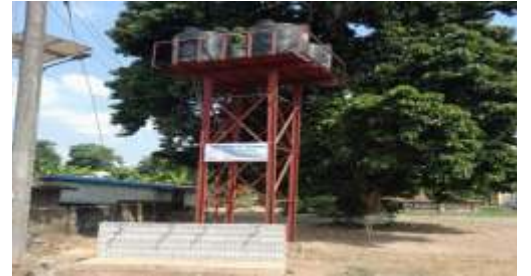
DRILLING OF WATER BOREHOLE WITH TANK AND STANCHION AT AKANU NDOKI VILLAGE IN IKWUORIE ATO IN NDOKI, UKWA EAST LGA
