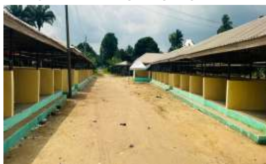
CONSTRUCTION OF FOURTEEN (14) BLOCKS OF TEN (10NOS) OPEN MARKET STALL AND RENOVATION OF TWO BLOCKS OF TEN (10NOS) OPEN MARKET STALLS AT AHIA ORIE UMUAJIOHA OBUZOR ASA COMMUNITY MARKET, UKWA WEST LGA
