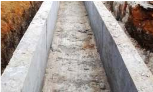
CONSTRUCTION DRAINS FROM OBEHIE TO AKWAETE BY UMUNTEKE ROAD JUNCTION TO UNUMKPO ROAD UKWA WEST LGA (2.4KM)
