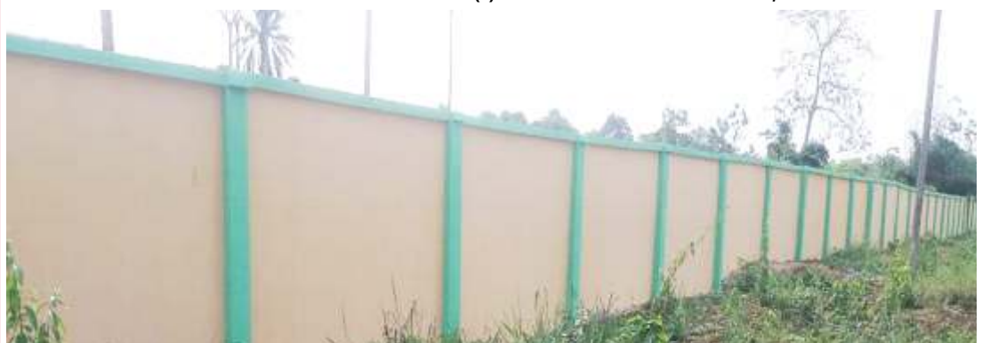
CONSTRUCTION OF PERIMETER FENCE OF OZAA SECONDARY SCHOOL (1.4KM), UKWA WEST LGA
