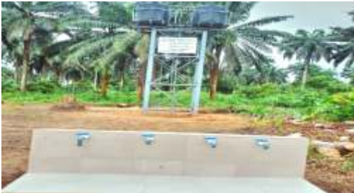
CONSTRUCTION OF WATER BOREHOLE AT UMUAKA, UKWA WEST LGA
