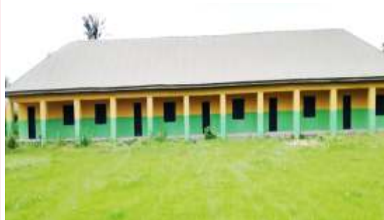
RENOVATION OF THREE (3) NOS. CLASSROOM BLOCK AT OWO ASA, UKWA WEST LGA
