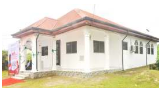
RENOVATION OF CRECHE FACILITY FOR NURSING MOTHERS AT HIGH COURT UMUAHIA NORTH
