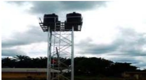
DRILLING OF WATER BOREHOLE AT OBAJI VILLAGE ISIALA NTEKE, UKWA WEST LGA
