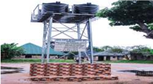
DRILLING OF BOREHOLE AND RETICULATION WITH TANKS AT UMUELECHI OBUZOR KINGDOM ISIMIRI, UKWA WEST LGA
