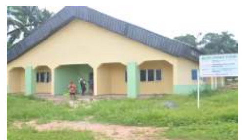
CONSTRUCTION OF UMUEZEGU HALL, NSULU, ISIALA NGWA NORTH LGA
