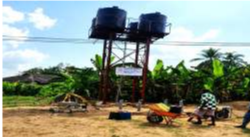
DRILLING OF WATER BOREHOLE AND RETICULATION AT ABAKI NDOKI, UKWA EAST LGA
