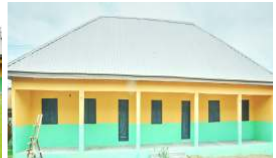
RECONSTRUCTION OF A TWO (2) CLASSROOM BLOCK AND TWO (2) OFFICES AT OBEHIE CENTRAL SCHOOL, UKWA WEST LGA
