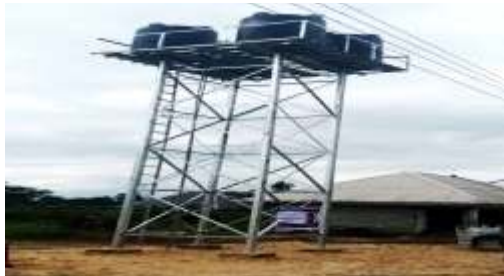
DRILLING OF BOREHOLE AT ASCENSION JUNIOR SEMINARY SCHOOL COMPOUND, UKWA WEST LGA
