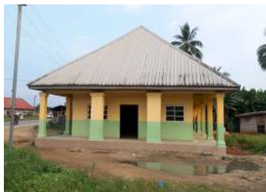
CONSTRUCTION OF UMUKWOR CIVIC HALL, UKWA WEST LGA
