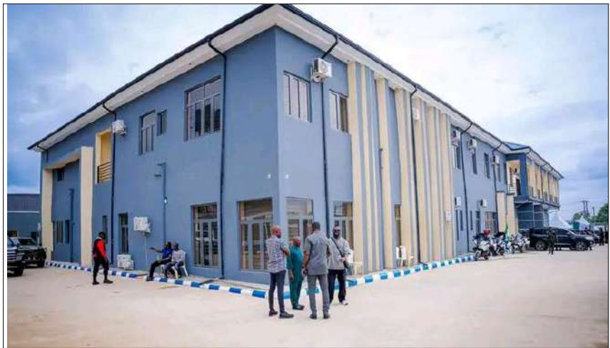
The newly built and furnished administrative complex of the Nigerian Air Force in Umuahia completed and officially handed over to the Nigerian Air Force by the Abia State Governor, Dr. Alex Otti.
