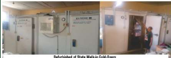
Refurbished of State Walk-in Cold-Room
