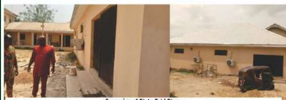
Demolition of State Cold Store
