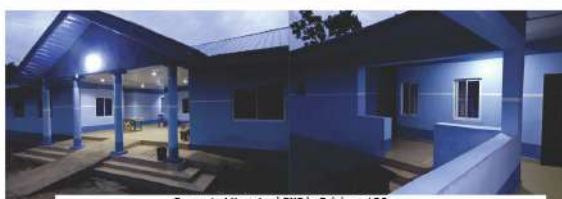
Renovated Ilimuhaci DHC in Paicima I/R&
