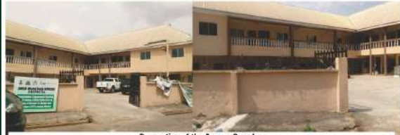
Demolition of the Banamu Penelau
