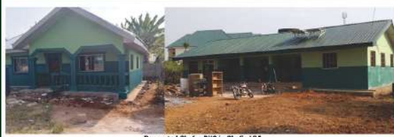
Renovated Okafor PHC in Ibafo I/R&
