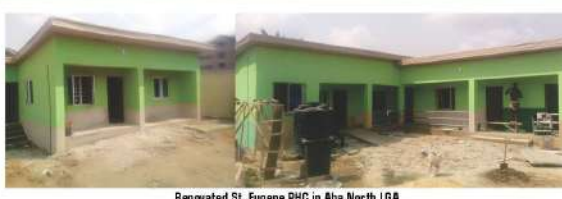
Renovated St. Eugene PHC in Aba North LGA
