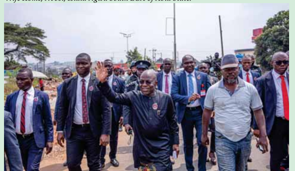
Gov Alex Otti of Abia State, during his inspection of the on-going reconstruction and expansion of Bank Road Umuahia, Abia State.
