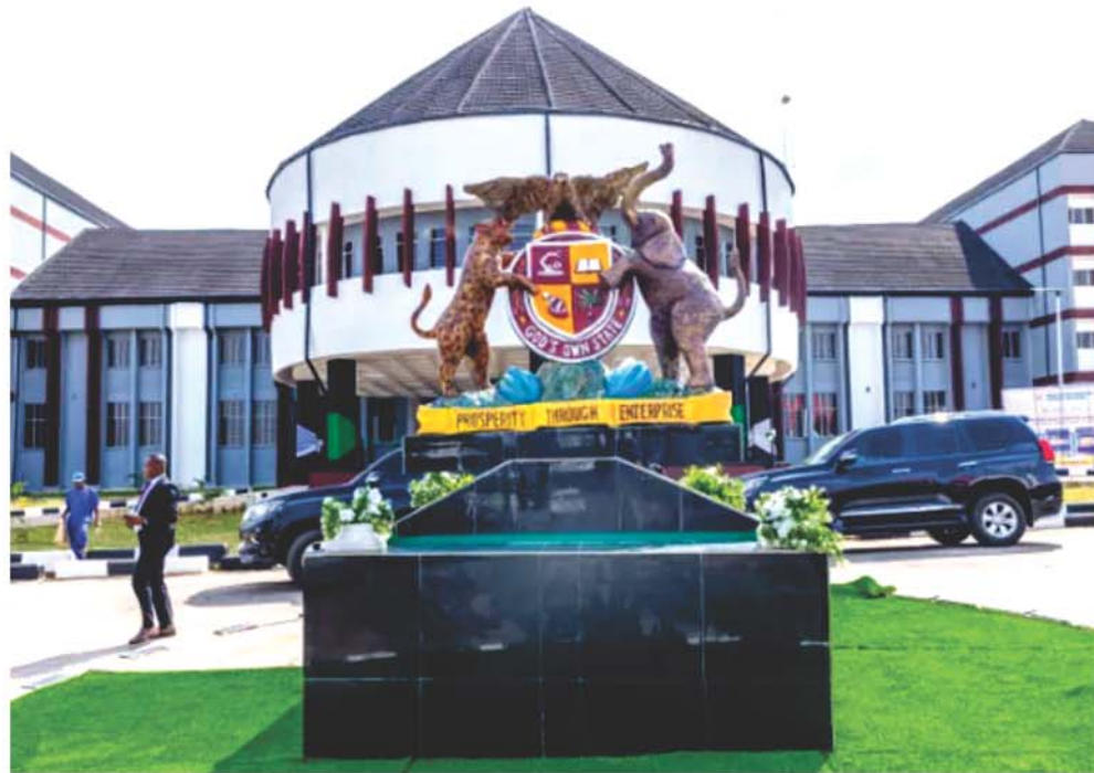
Newly Retrofitted Nnamdi Azikiwe State Secretariat Complex
