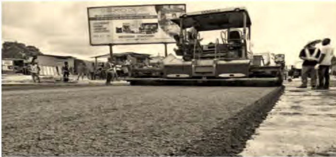
■ Road construction work in Abia by Gov. Alex Otti's government, recently.
