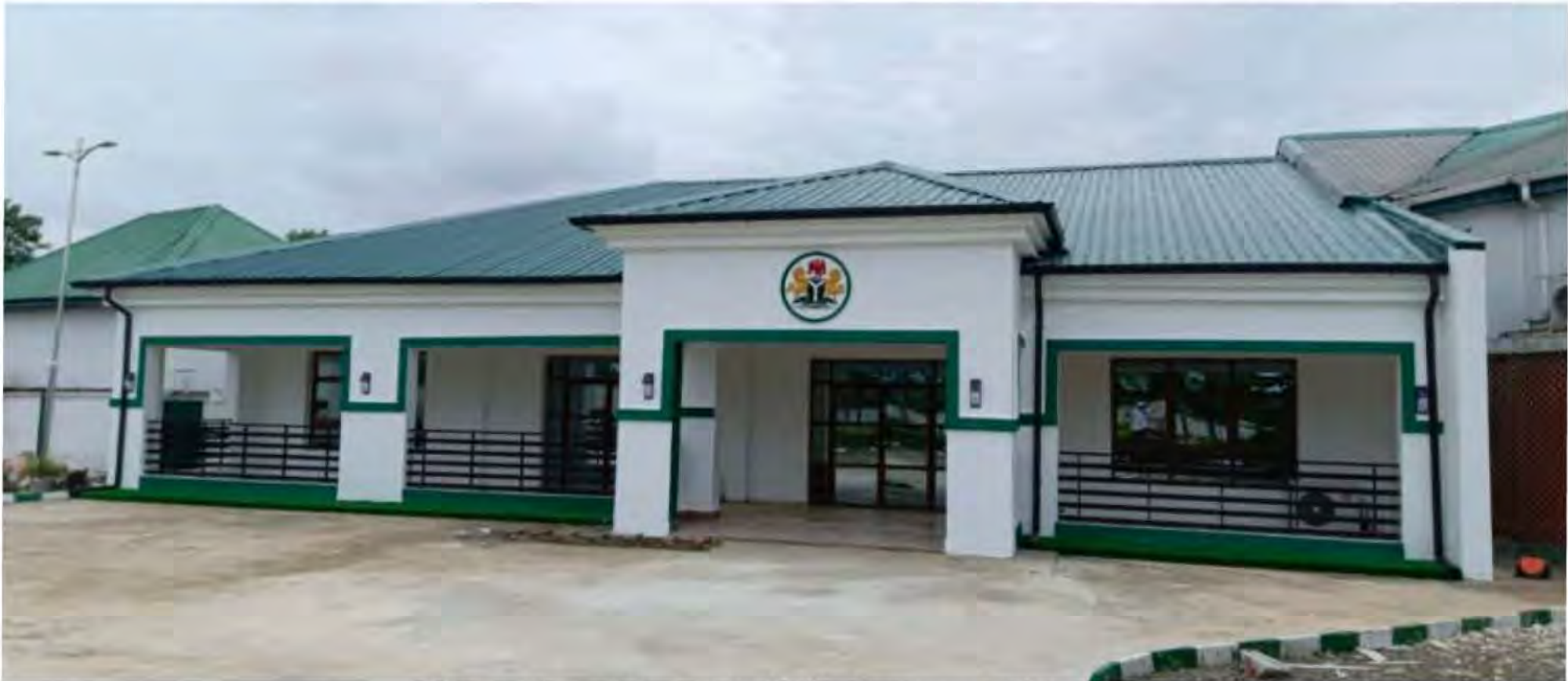
Renovation of Banquette Hall - Government House
