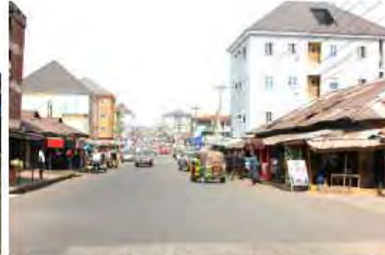
■ Uzuakoli Road, Umuahia after maintenance
