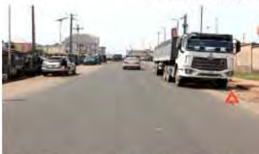
■ Uwalaka by shoprite Umuahia after maintenance
