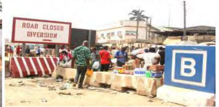
■ No. 1 Portharcourt Road Aba
