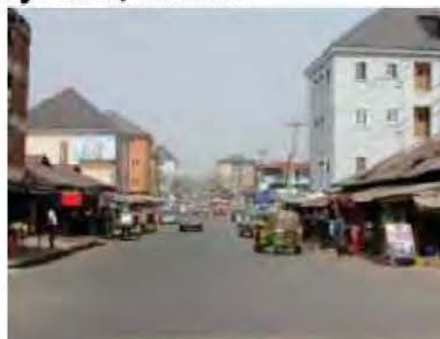
■ Uzuakoli Road, Umuahia after maintenance
