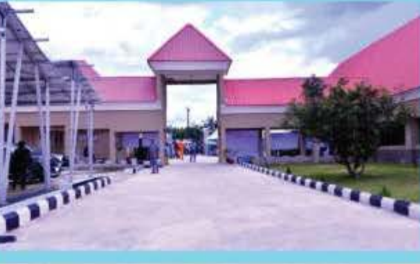
14. Entrance view of the Amachara General Hospital Umuahia.
