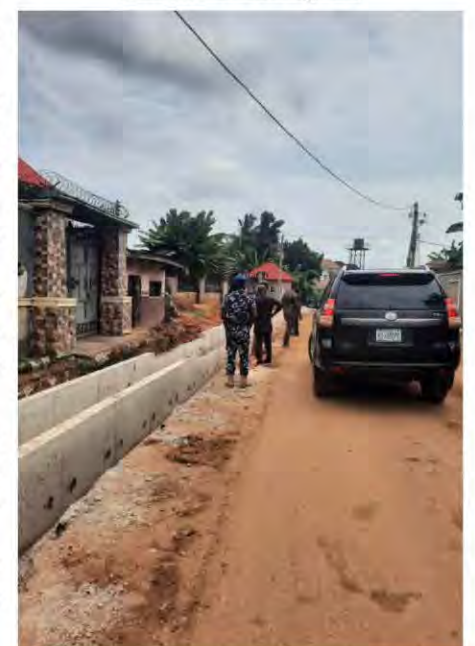
■ One of the roads under rehabilitation
